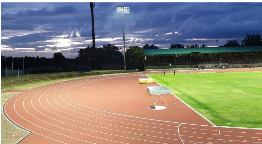
Figure 9: The renovated Coetzenburg athletics stadium.
